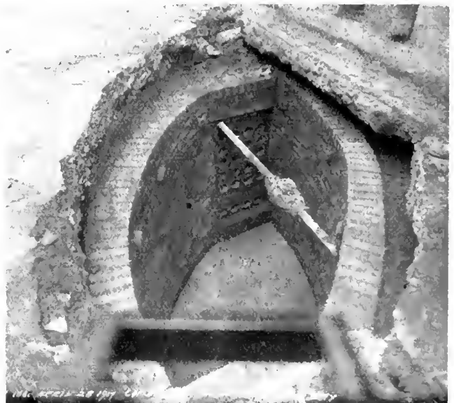
Fig. 3—Offset manhole changing course 4 ft. to right.
